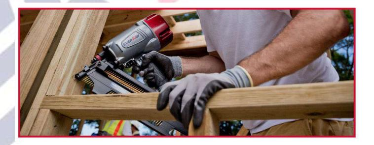
A framing nailer can use coil nails, as well as strip nails. See EVERWIN's prior article "A Comparison between Coil Framing Nailers and Stick Nailers".
